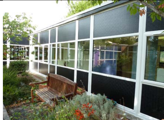
Clovenstone Primary school – New windows
