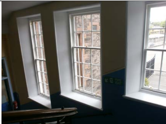
Abbeyhill Primary school – window refurbishment
