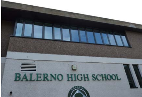
Balerno High School Replacement – New windows
