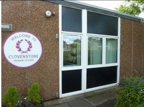
Clovenstone Primary School – New Windows
